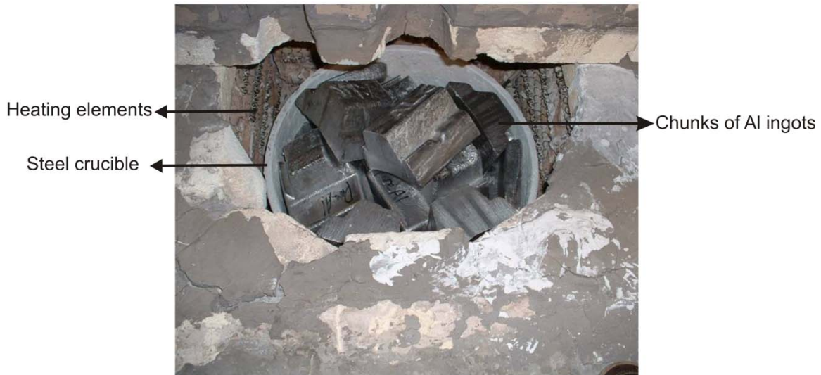
Figure 1 - The electrical resistance furnace including the revolving liquid metal tank showing the Al charge prior to melting
